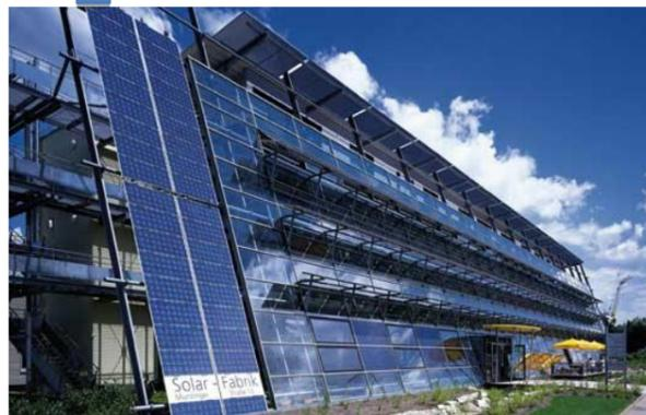
Figure 1: Building Integrated PV coupled with DHW (Auzenet, et al 2013)
