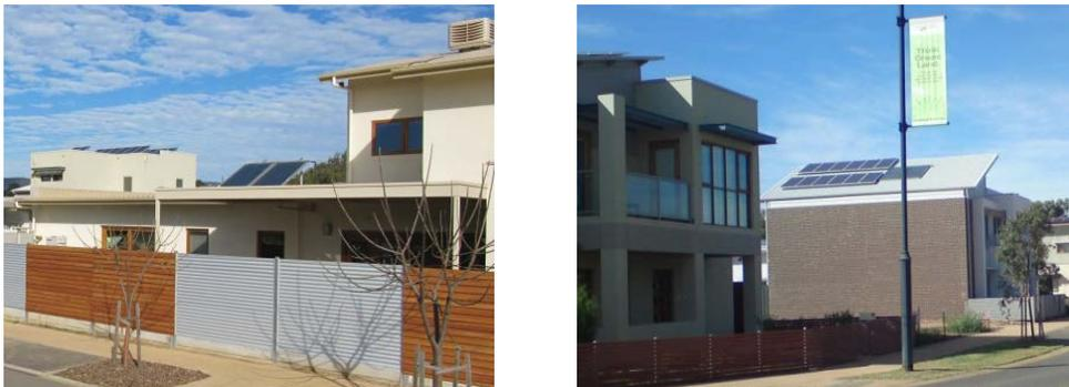
Figure 4 Examples of Lochiel Park houses showing integrated solar technologies
